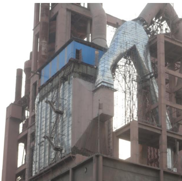
Replaced L-1 C line ESP by Baghouse
