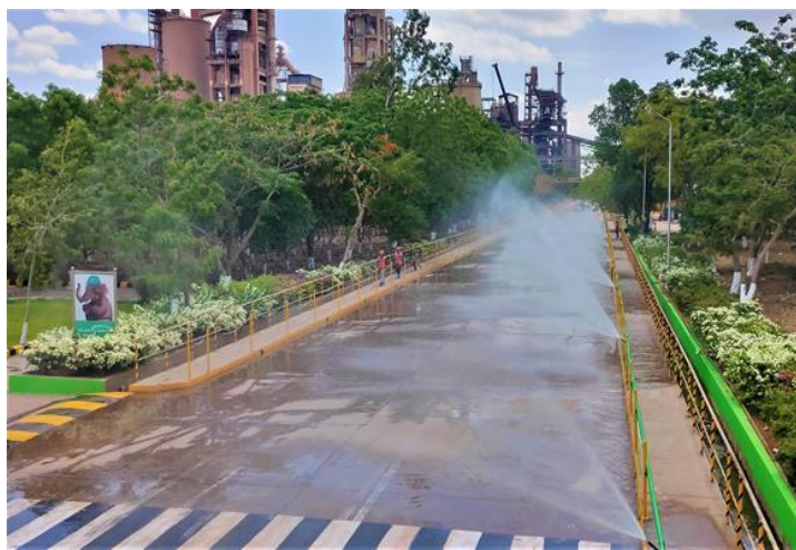
Automatic water sprinklers/Rain guns at Plant Road
