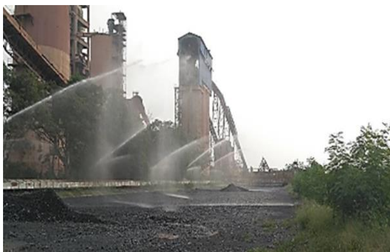
Rain guns at Limestone stockpile
