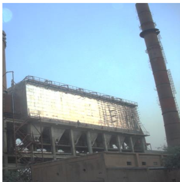
Replaced L-1 K line ESP by Baghouse
